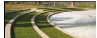
Post-Installation: Burrow-free and erosion-free
