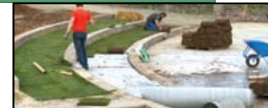
Installation of XCLUDER GEO
