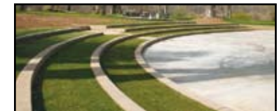
Post-Installation: Burrow-free and erosion-free
