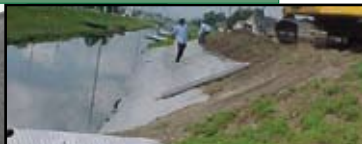
Installation of XCLUDER GEO
